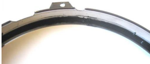
RTV in mounting ring
