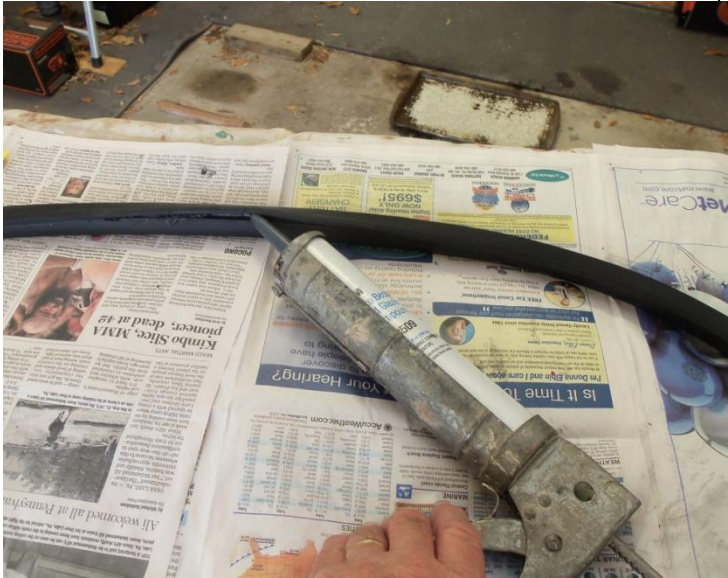
Applying sealant all the way around the inside of the gasket.
