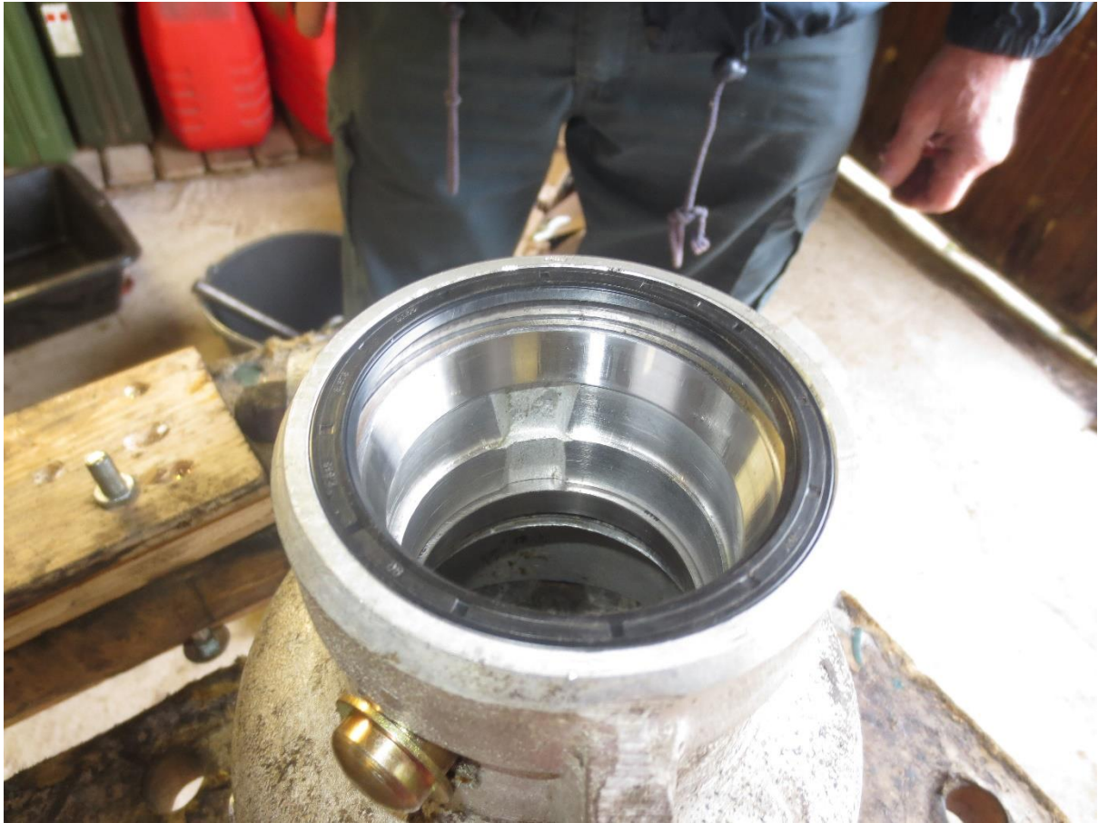
Photo 17: the new bearings' outer races in place in the clean carrier. Note the outer bearing's oil seal has to be installed at this point, as shown in the photo. Now the hub has to be fitted to the carrier. First the new outer bearing, inner race is driven onto the hub, see photo 18.
