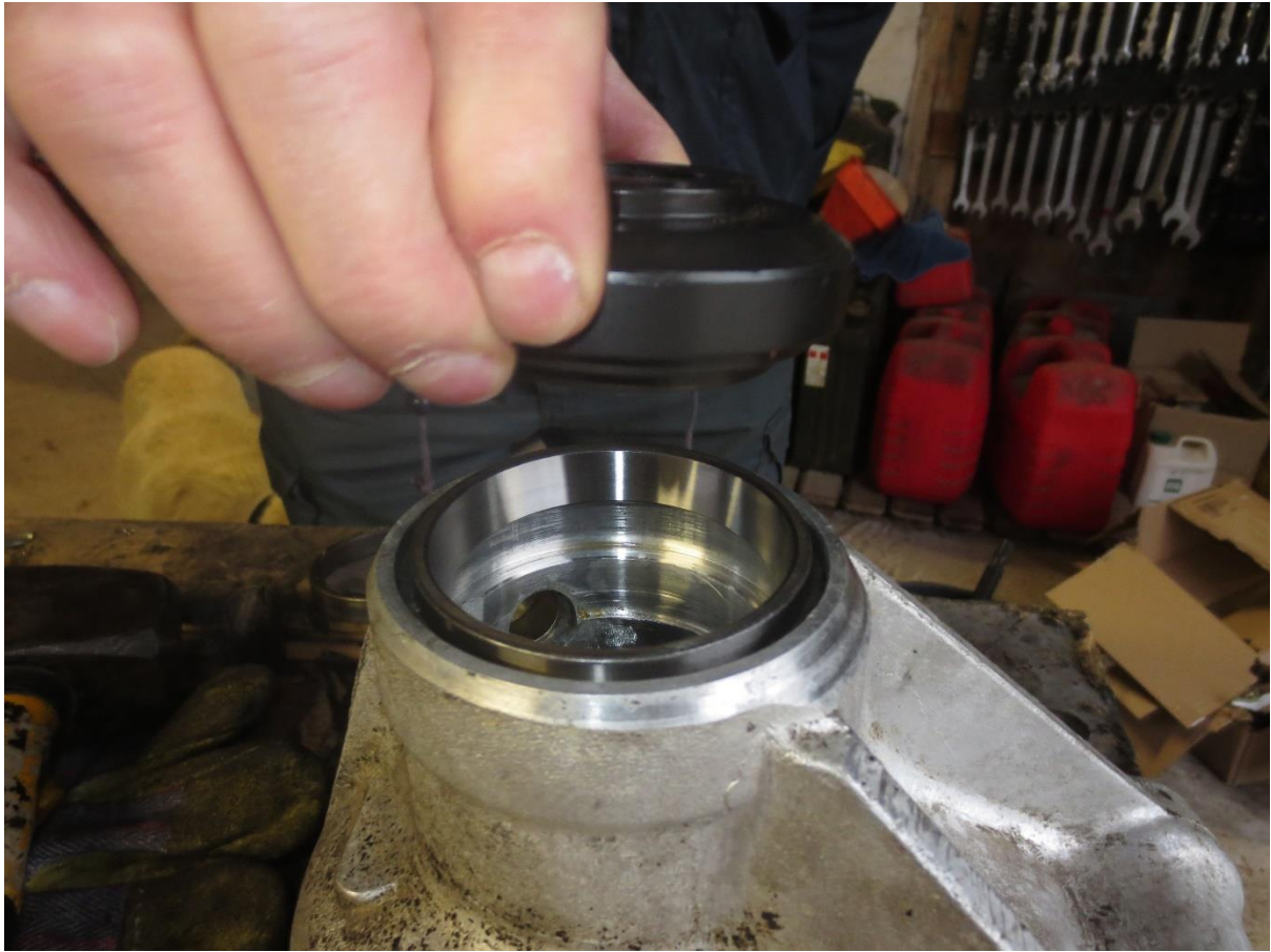
Photo 15: the new outer bearing race being driven into the carrier.
