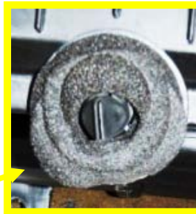
Duck bill Hose showing through the sealing material that seals between the AC Drain hole and the vehicle firewall.
